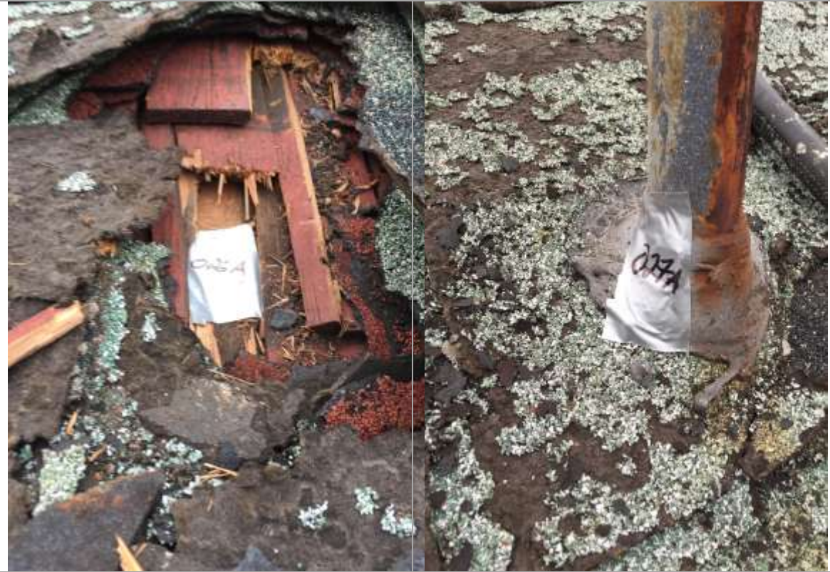
027A-Roof Vent Mastic (5% Chrysotile)
