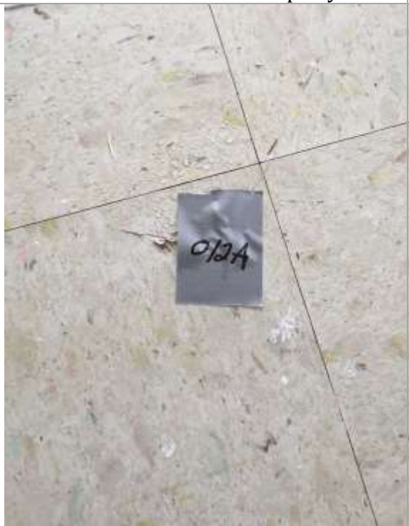
012A-Bedroom 2 Top Layer Flooring (3% Chrysotile)
