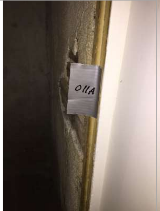
011A-Exposed Plaster Closet
