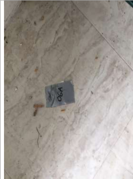
06A-Front Entry Flooring
