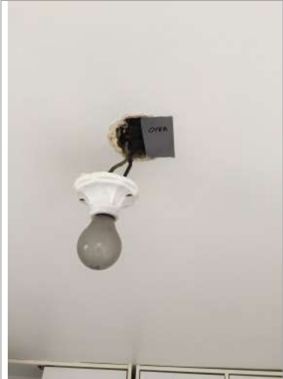
018A-Electrical Cable Insulation
