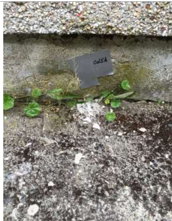
028A-Foundation Wall Mortar
