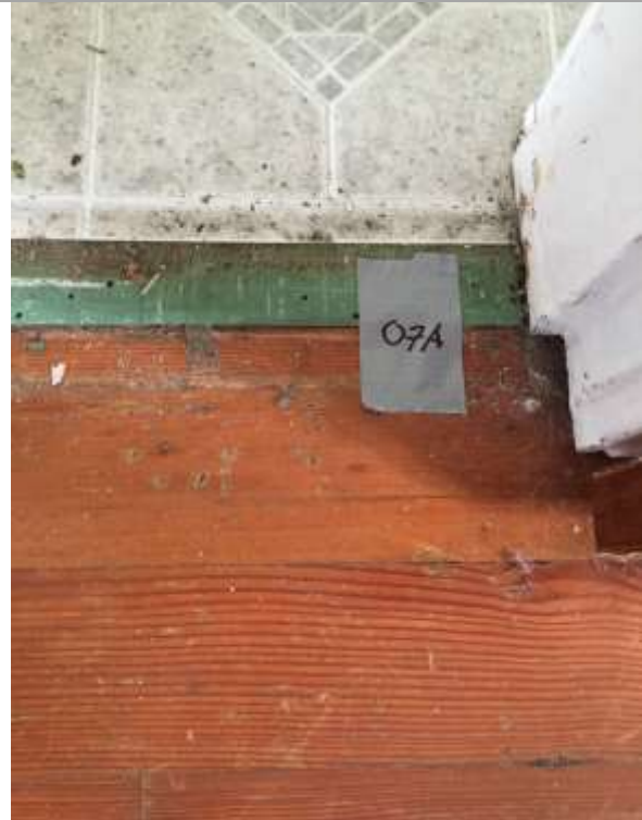
07A-Bottom Layer Flooring hallway (2% Chrysotile)
